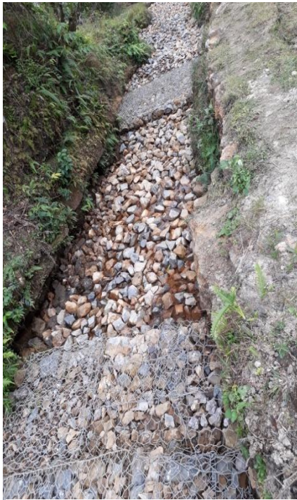
Fig. 5.2a: Photograph of an open limestone Channel 2
